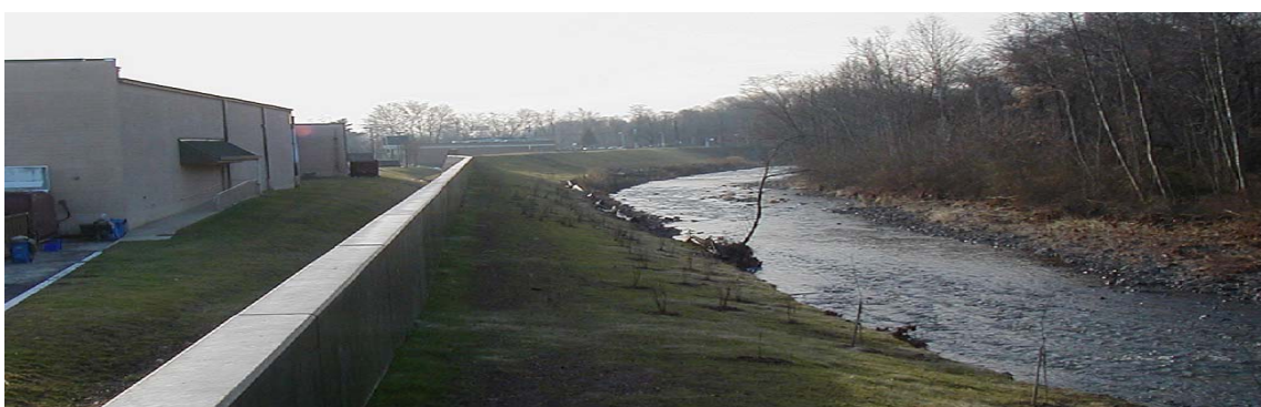
Floodwall along Middle Brook in Somerset County
